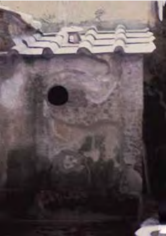
IMAGE 71 An ancient home contains a hole in the wall of the kitchen area. This was an early form of ventilation.
