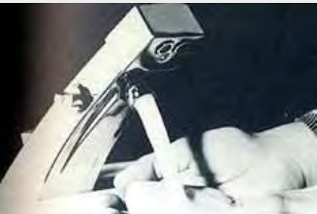
IMAGE 84 Automatic washing machines. The faucets are activated by a sensor for hands-free operation.
